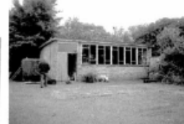
EXISTING PLANT ROOM, OIL STORAGE & GREENHOUSE - to be demolished
