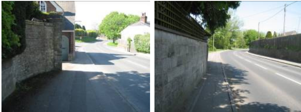
Figure 7 Narrow sections of existing footway and potential conflict points.
