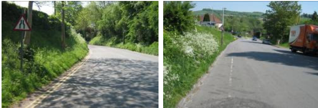
Figure 3 Narrow carriageway and Railway Bridge.
