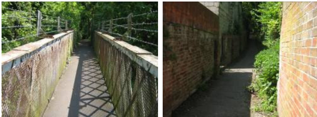
Figure 6 Milford Hollow - bridge and foot path.
