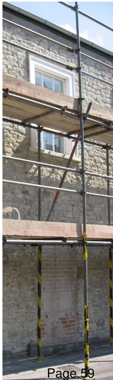
This doorway was blocked up with red bricks, possibly of circa 1900 Gillingham origin, and this is not referred to in the application; the applicant has removed these and replaced with some new non-matching stone.
