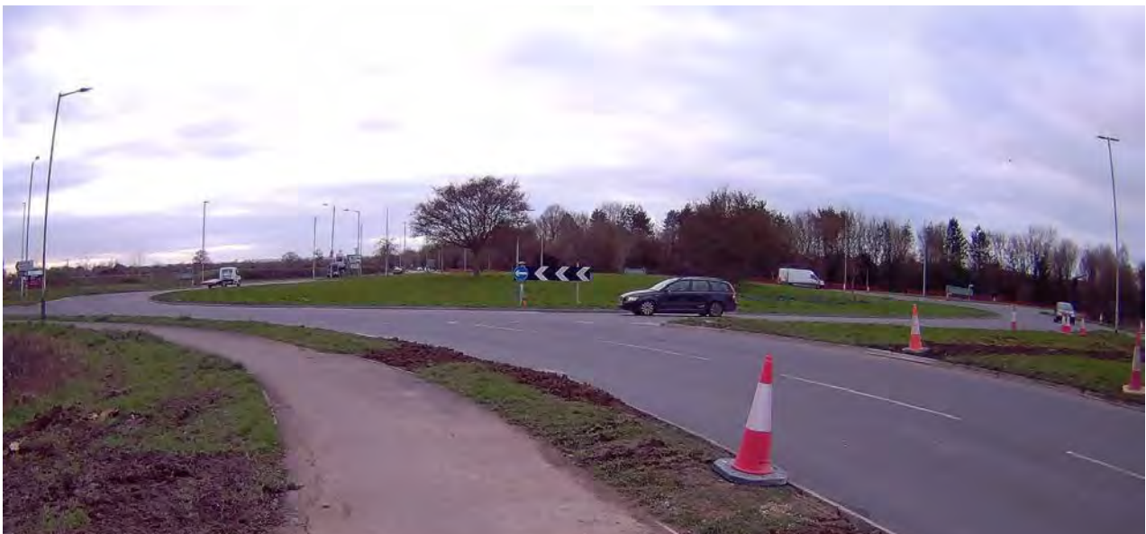
(View 4 – Bowerhill roundabout from A365, Pathfinder Way to left, Spa Road to Town, right.)
