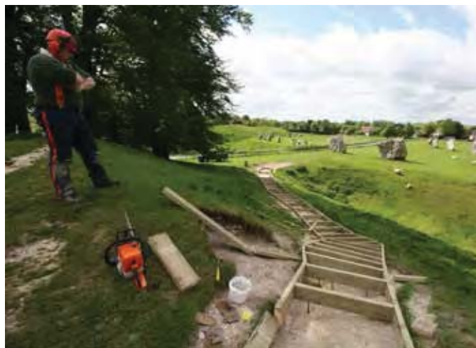
'Drapes' laid over the monument to protect it from erosion by visitor footfall
