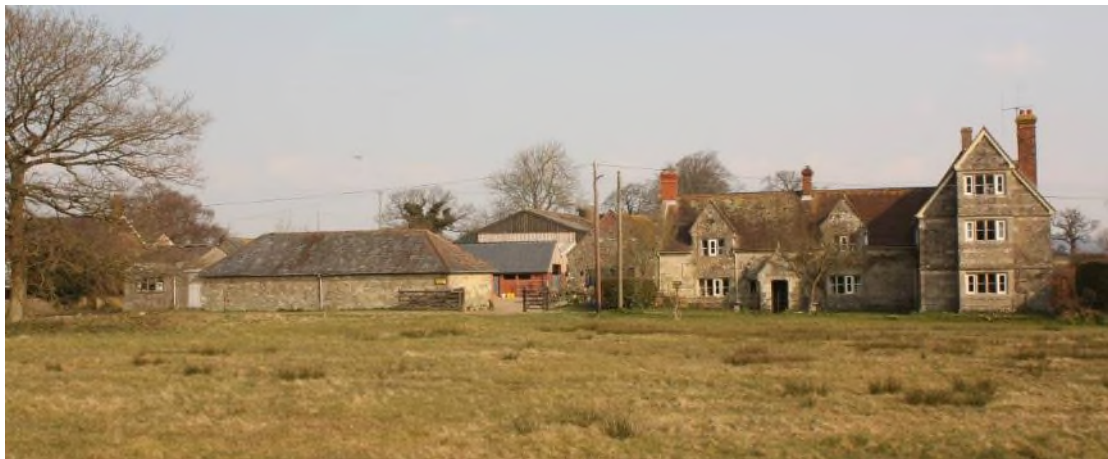
Figure SY5 Church Farm over-looking Church Green. The lower part of the farmhouse dates from the 16 th century and was enlarged in the 17 th century. The farm buildings all appear to date from the 19 th century and formed a courtyard group with an L-plan element and other detached buildings.
