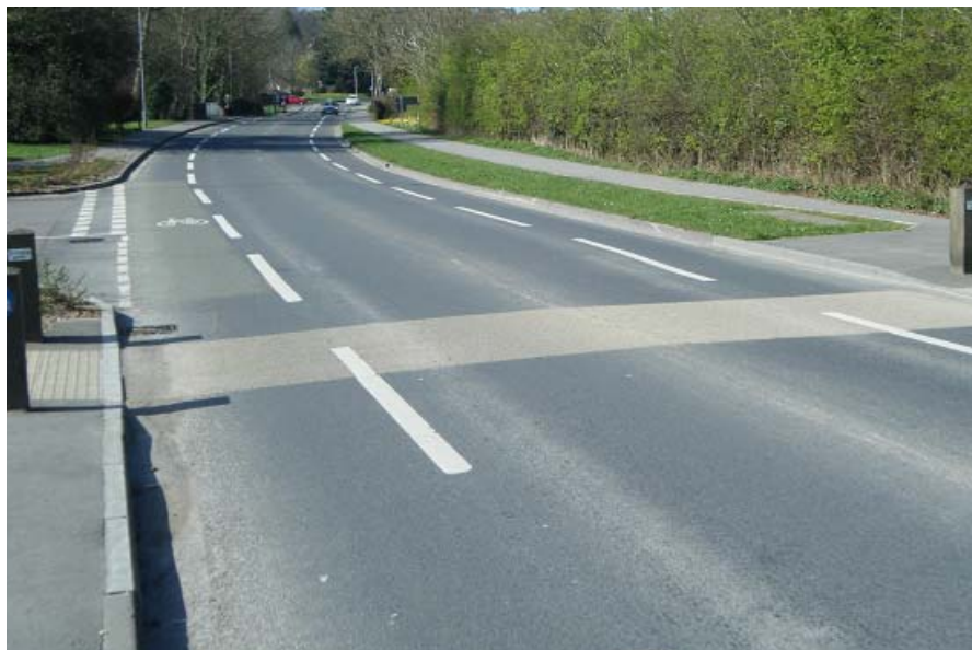
Picture 7.4 Removal of centre line with cycle lanes, Laverstock
