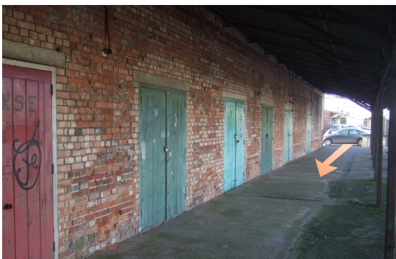
Image 3: Pedestrian route from station past former station building - potential commercial units
