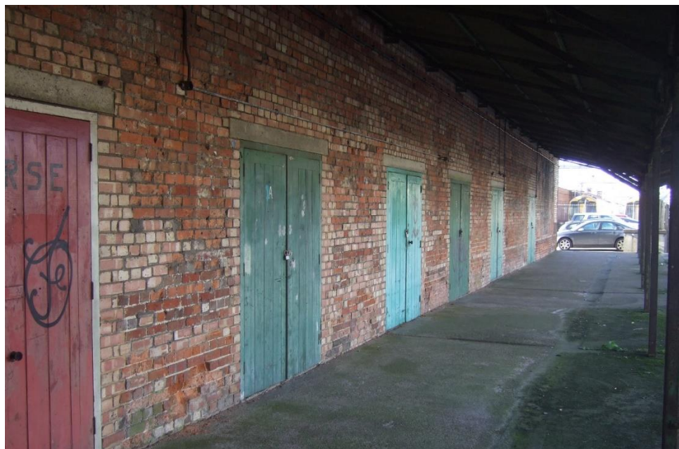
Figure 6-2 Route to new entrance past unused part of Former Station Building
