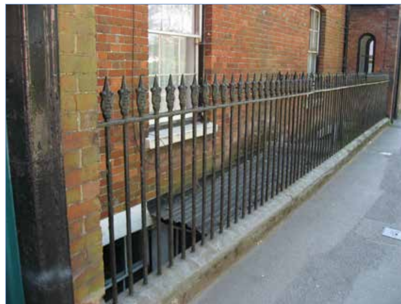
Fig 84 Cast iron railings
