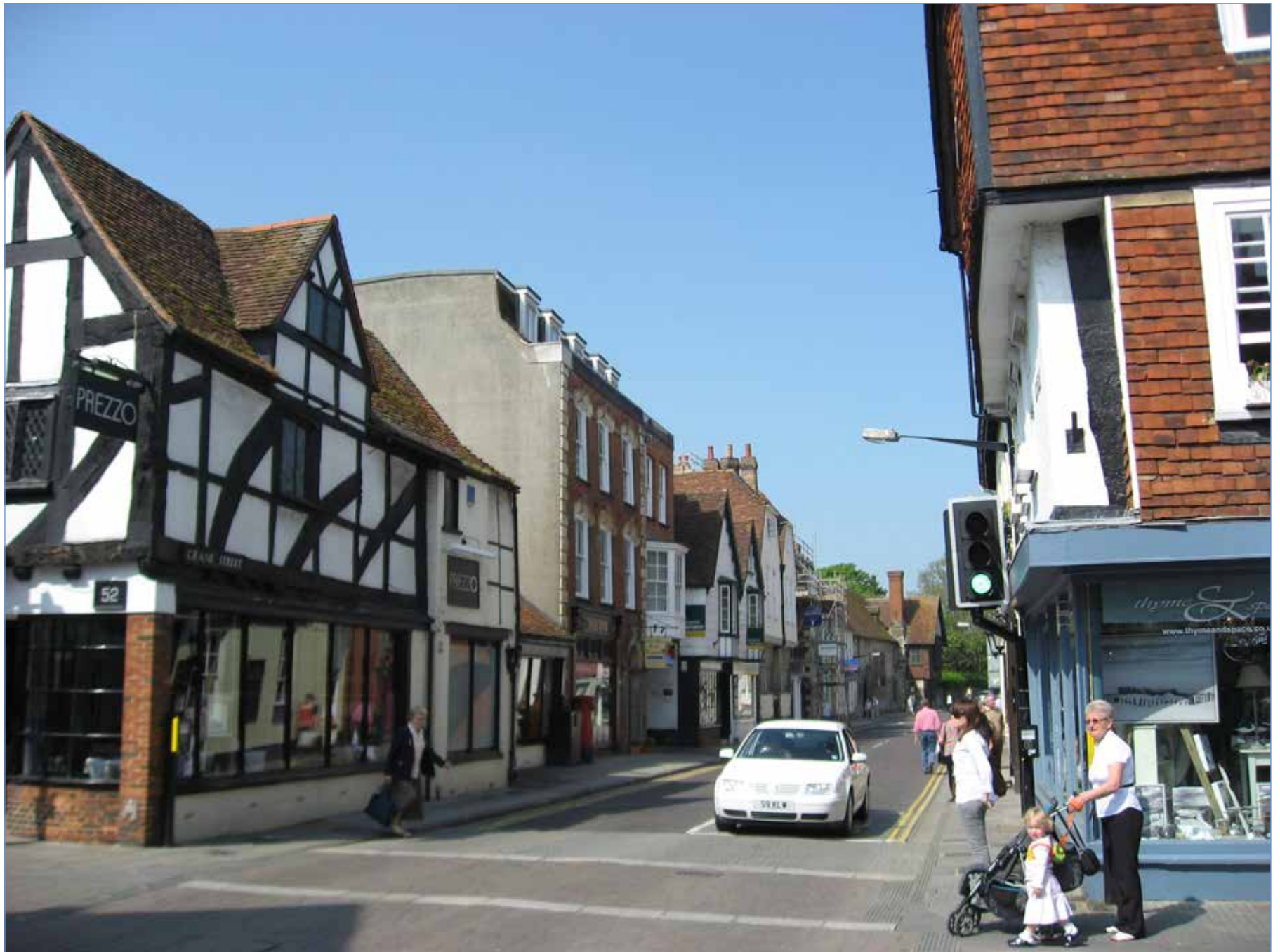
Fig 53 Crane Street, south
