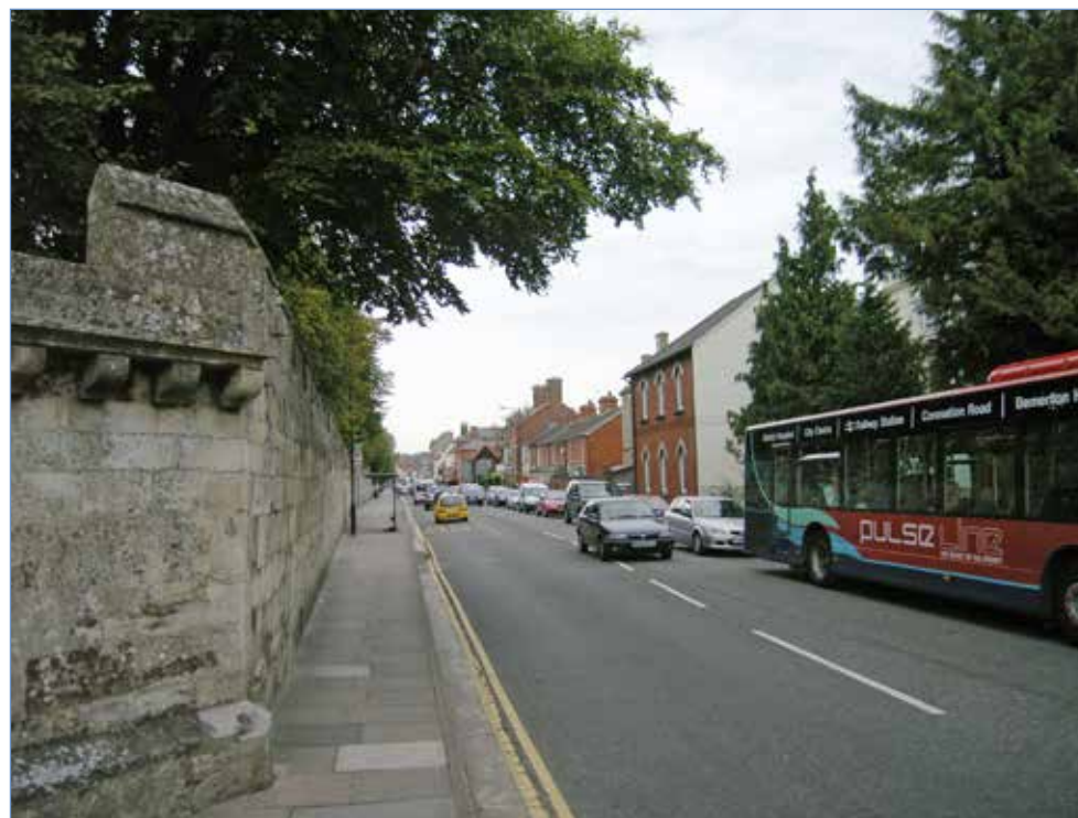
Fig 70 View of Close wall from Exeter Street
