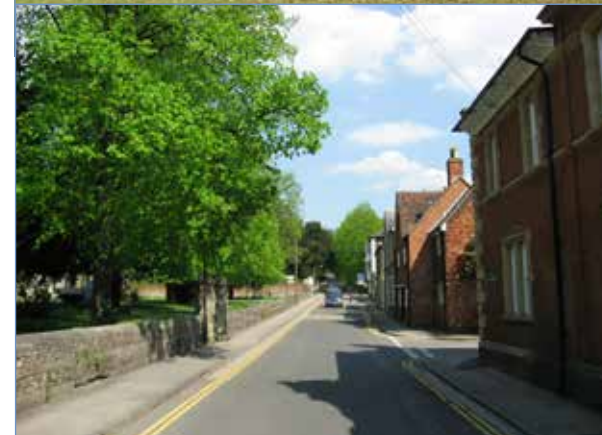
Fig 73 Loss of railings
