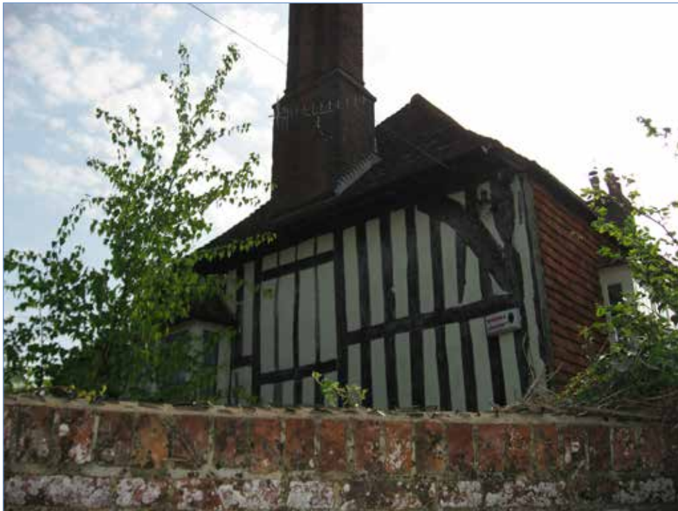
Fig 102 Timber framing, Harnham Road
