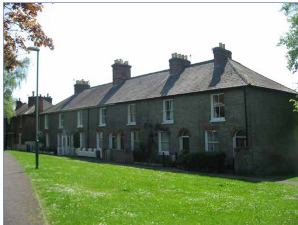
Fig 51 East of Greencroft Street
