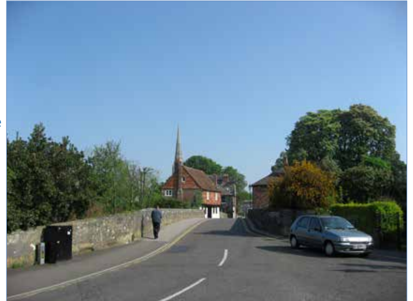
Fig 99 Harnham Road and the southern side of Ayleswade Bridge
