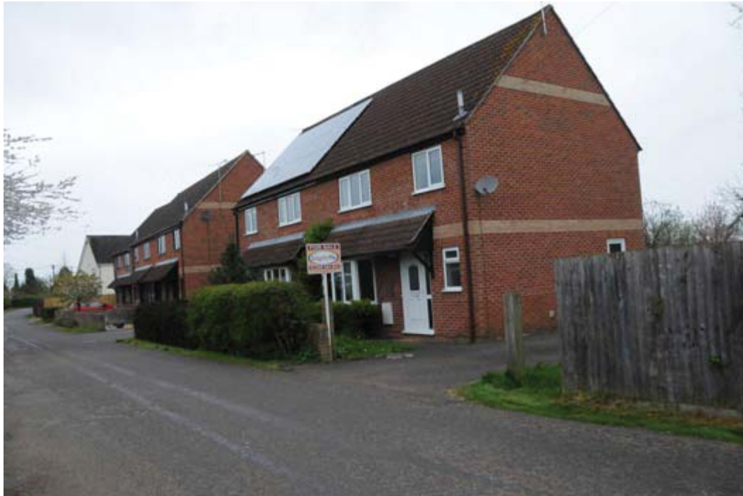
FIG8: Housing adjacent to site HS1 – set 4.5m back from the edge of the road
