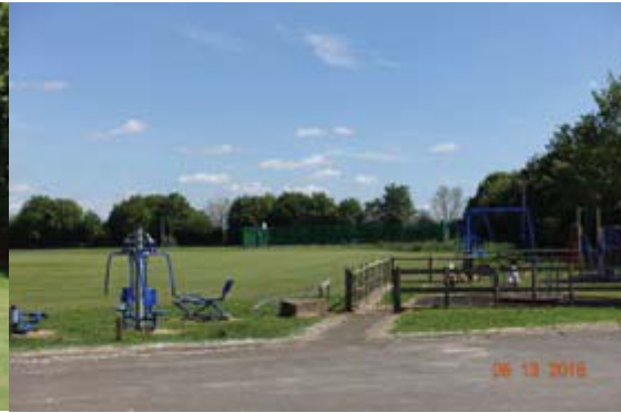
FIG2: Part of the Recreation Ground with play facilities and the multi-use games area to the rear
