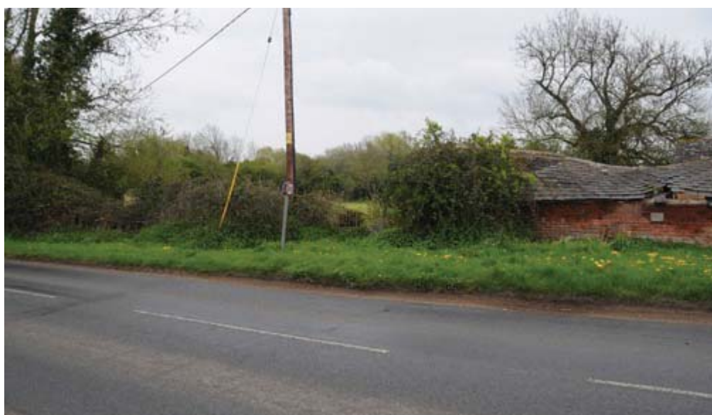
Pic 17: Site HS5 and associated dilapidated buildings
