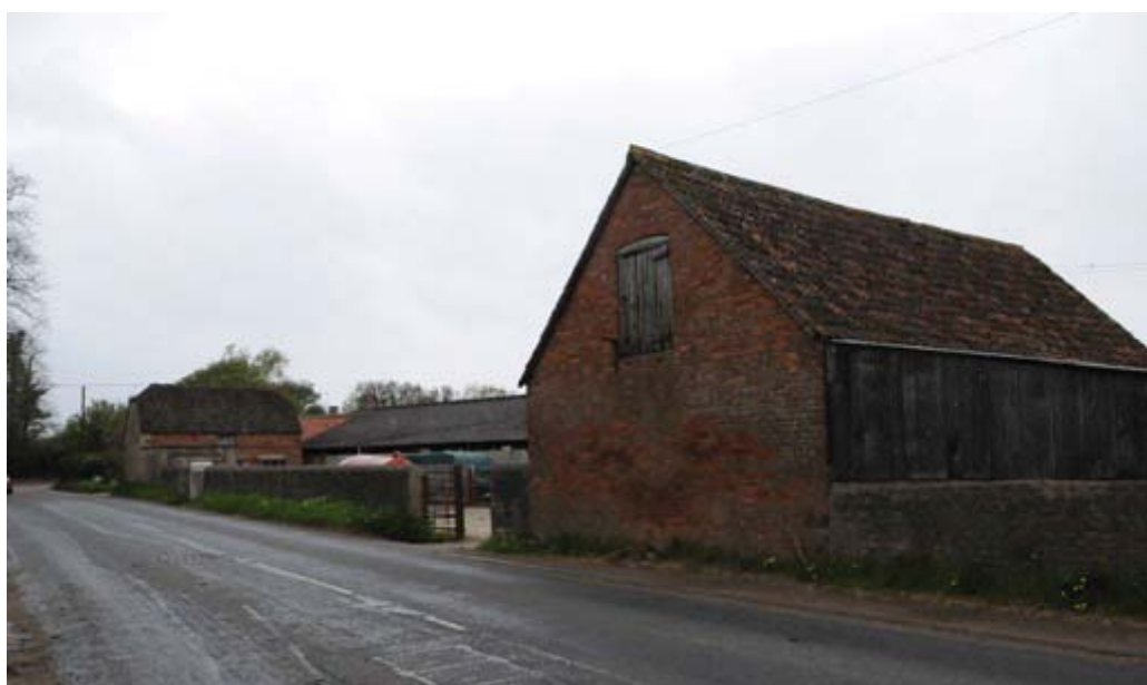
Pic 14: Site HS4 from the east
