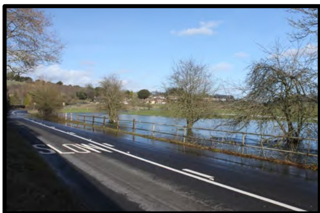
River Bourne overflowing on to the main A338 Trunk Road North of Hairpin Bend at Idmiston
