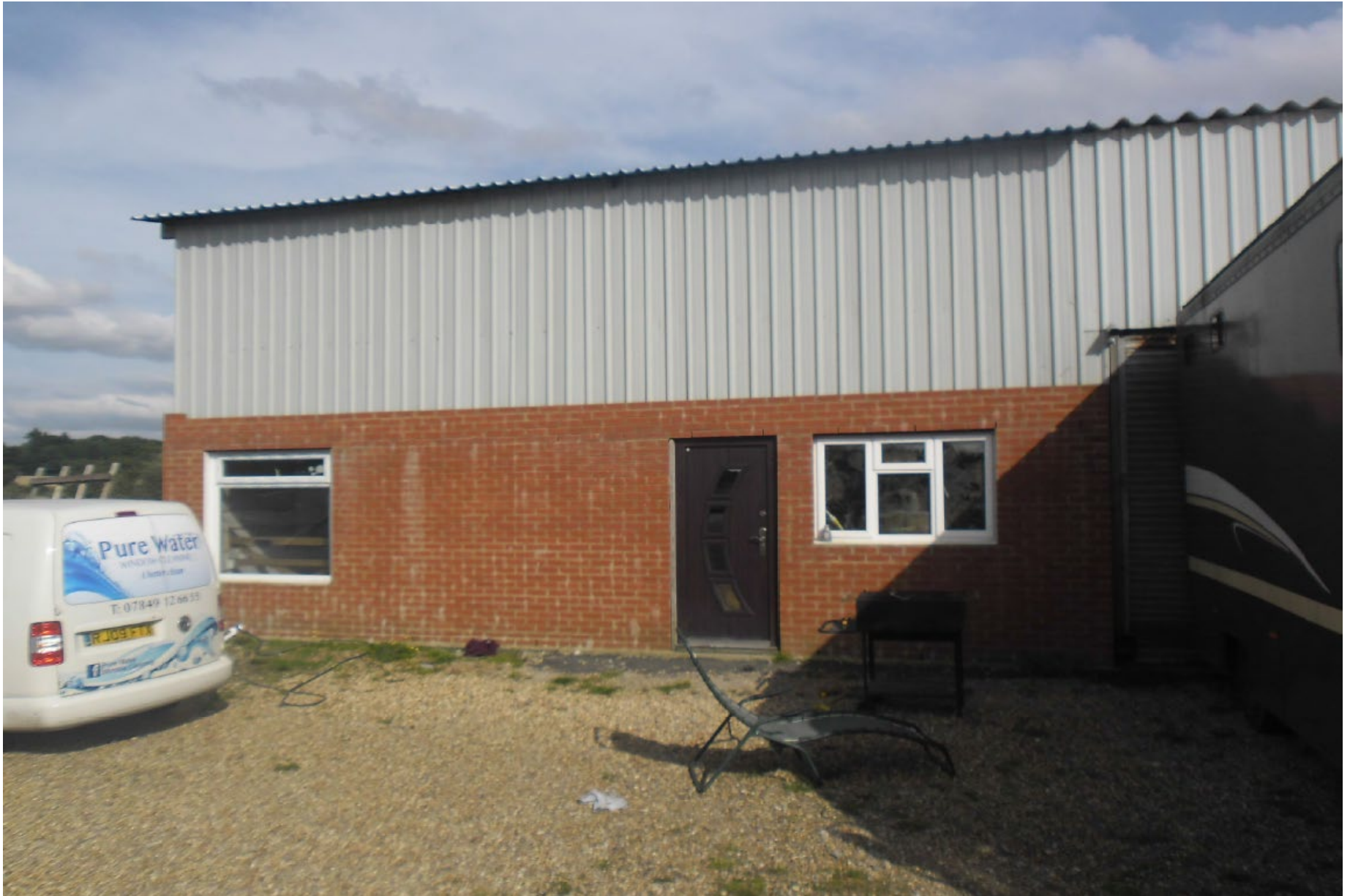
Existing side elevation (West) of Barn
