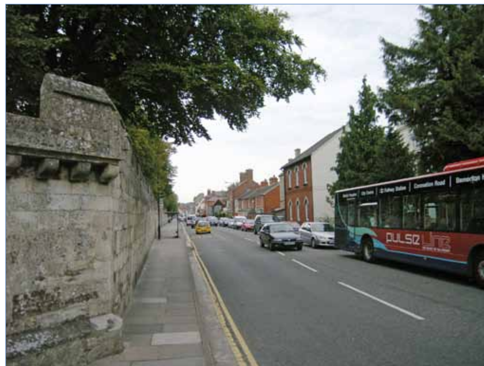
Fig 70 View of Close wall from Exeter Street
