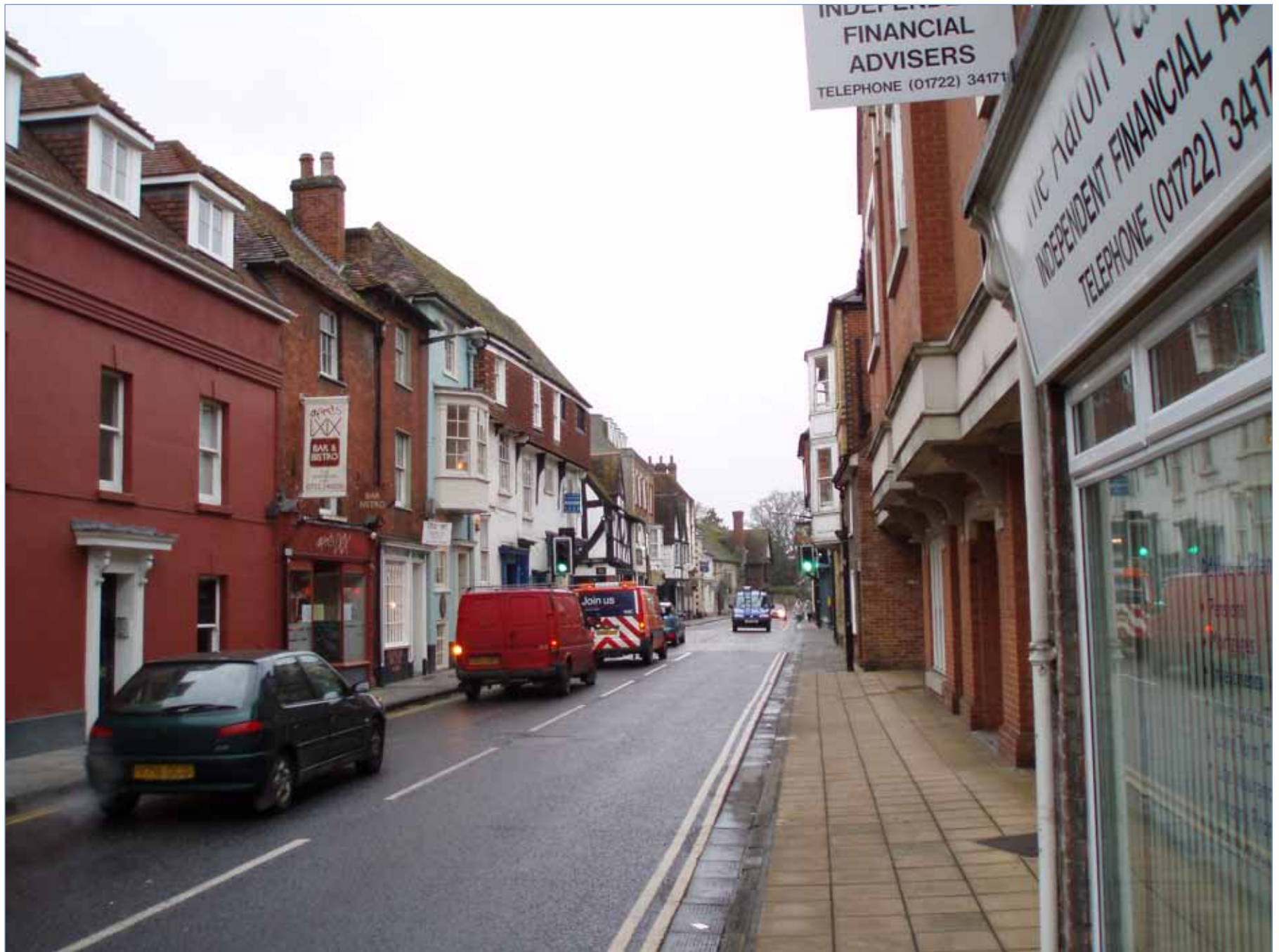
Fig 55 New Street, south
