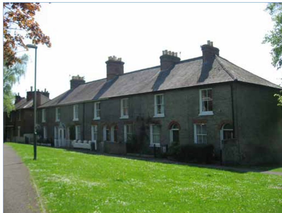
Fig 51 East of Greencroft Street
