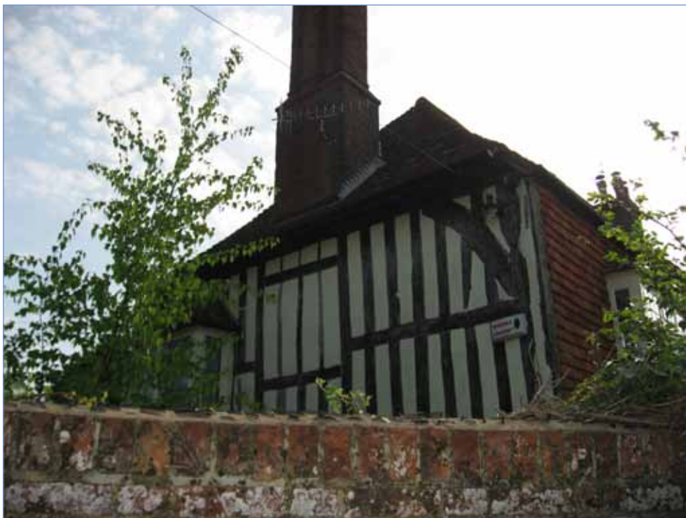
Fig 102 Timber framing, Harnham Road
