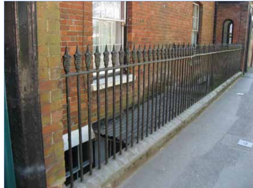
Fig 84 Cast iron railings
