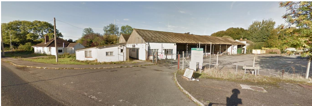
View of application site from Furnax Lane
