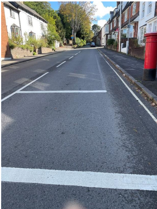
Image 1. Advanced stop line - front view
