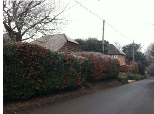
Existing Garage from Road
