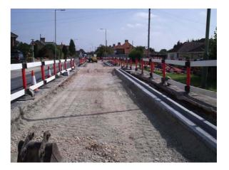
At Salisbury the second phase of works on the A3094 Netherhampton Road completed work started to the reconstruct this section of road in 2005/6. On the A3102 at Sandridge Hill, east of Melksham, a major maintenance scheme included improvements to forward visibility to bends on the hill, kerbing of the carriageway and improved drainage.
