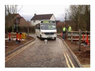
A scheme to install a rising bollard to provide a bus only access point was completed at Bumpers Farm, Chippenham. The bollard is controlled by a roadside card reader and allows a new bus service to be provided to this important employment area. This is the first rising bollard using this technology to be installed in the County.
