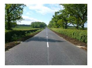
The second phase of major reconstruction work on the B4696 at Leigh in the very north of the county was completed. This route was suffering heavy rutting caused by quarry lorry traffic and poor ground conditions. The scheme provided improved surface water drainage and new kerbing at key locations.
