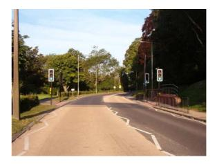
The junction at Stoney Gutter on the A350 near Trowbridge was altered to allow the right turns from the main road to be signalled separately. This should improve safety at the junction by reducing confusion to drivers waiting to turn right. The design of a new signalled junction at Bradford Leigh incorporating pedestrian facilities has been completed.
