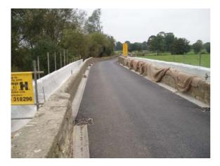
Mouchel Parkman was responsible for the design and supervision of a contract for extensive stabilisation work to the gravity dam of Braydon Pond, an ornamental lake near Malmesbury. The county road carried by the dam had been closed for an extended period due to a slip in the face of the dam. Work comprised piling, regrading and vegetation control followed by the complete reconstruction the of carriageway.
