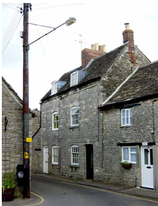
Fig 19: The Horsefair is spoilt not only by parking but also by unsightly overhead wires and poles.
