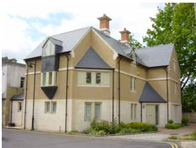
Fig 8: Recent infill in the heart of the Conservation Area close to the Abbey
