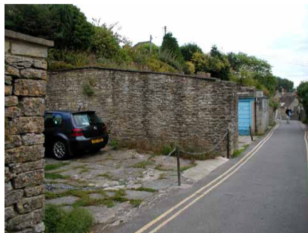
Fig 27: Modern garages, car spaces, cables and poles all intrude into the historic ambience of the area.
