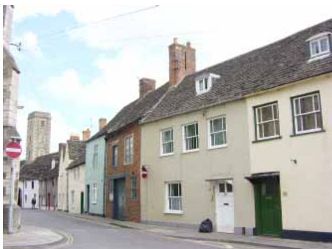
Fig 4: The view to the tower of Tower House from Cross Hayes is degraded by the unsightly overhead wires and signage
