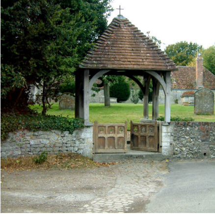
There is little formal paving in Wilcot. This section of setts was presumably laid to provide the vicar of the time with a dry route from the church to the vicarage.
