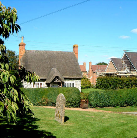
Rose Cottage is an important component of the group of buildings fronting the churchyard. The overall design of the building, its scale and proportion form a complete picture which needs to be preserved unaltered. Thatch is the traditional long straw.
