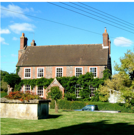
The front of Manor Farmhouse is an attractive representation of 18 th century style building incorporating high quality brickwork, double-hung sash windows and a simple roof form with gable end chimney stacks.
