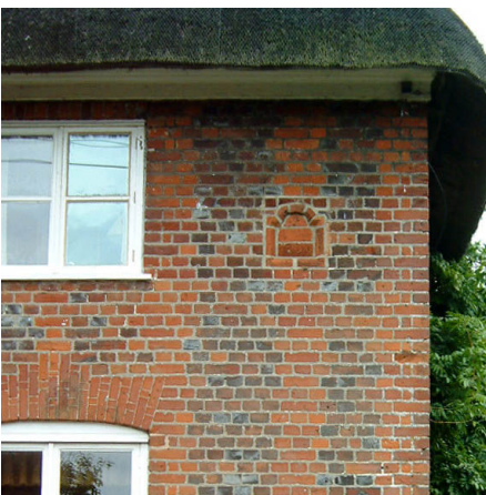
The brick front wall to Paradise Cottage is laid in an unusual header bond with overburnt blue brick selected to create a distinctive vertical pattern. The rubbed brick recess carries the date 1729.
