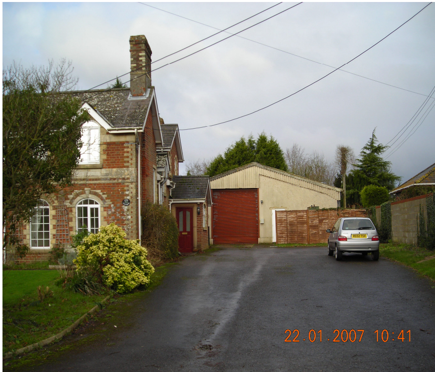
Site – looking from road
