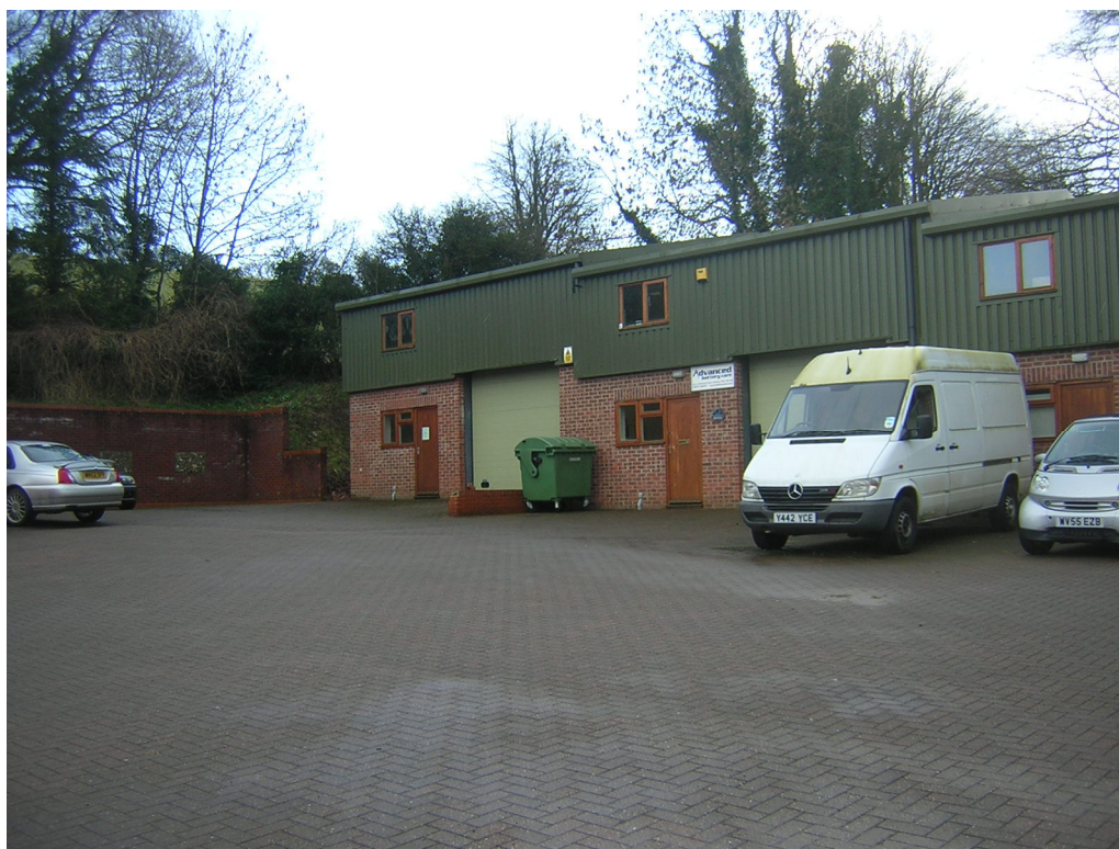
Picture of site – the unit concerned is the one at the left of the picture
