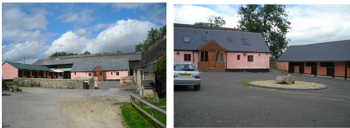
The application site
