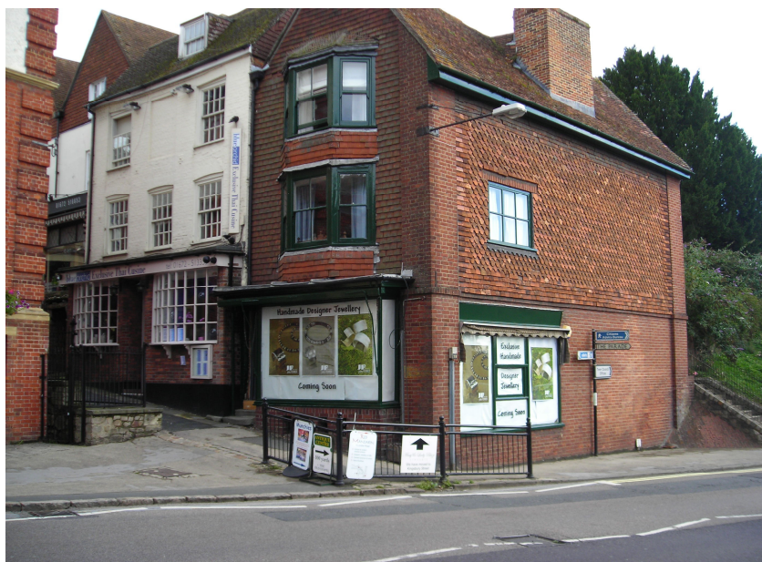
Existing building – the shutters would be set back from the shopfronts
