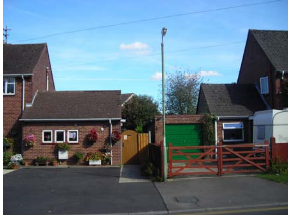
The site – the single storey extension and garage behind the five-bar wooden gate
