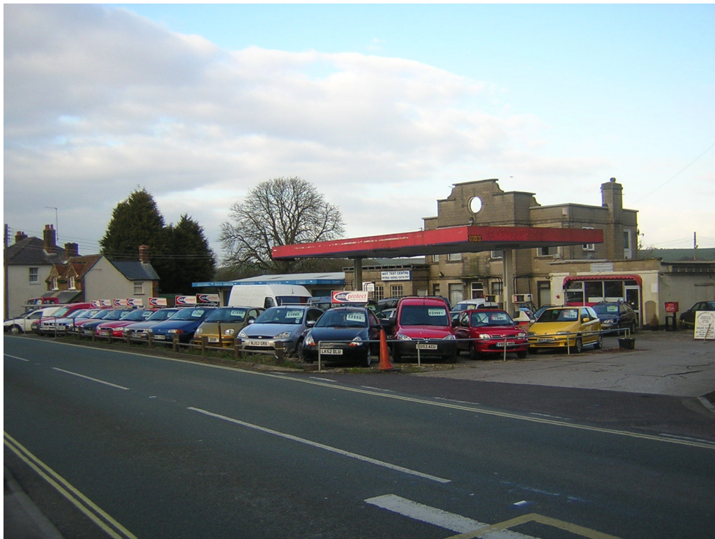
Photograph 2 - Garage site from south
