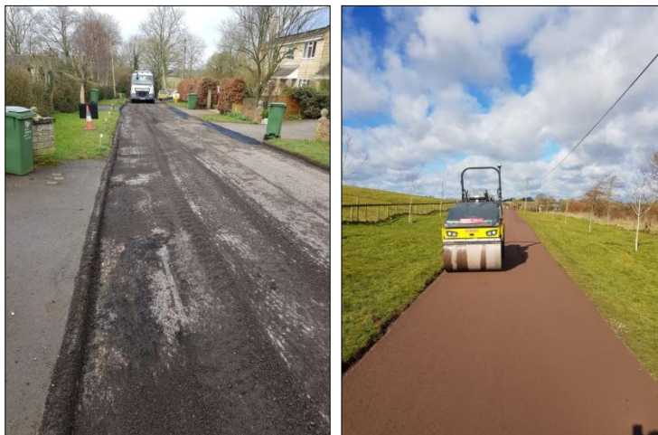
In-situ recycling makes use of the existing road material by excavating and mixing it and treating it to increase its strength
