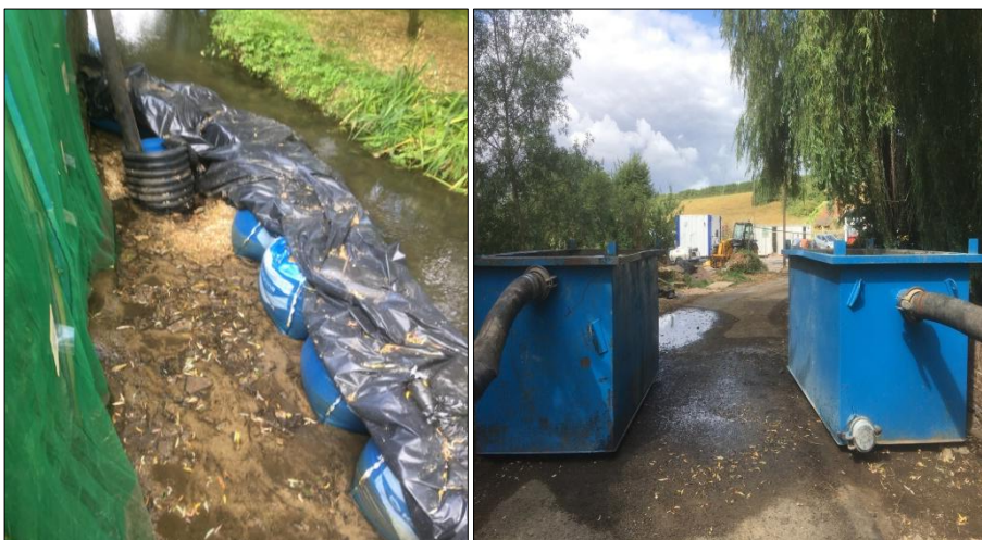
Filtration tanks can be used as part of the over pumping operation
