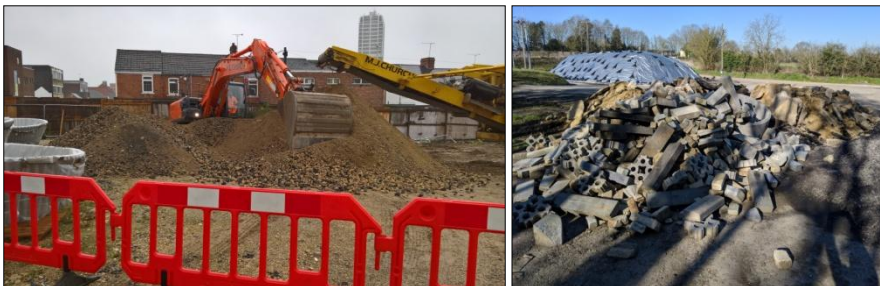
Waste concrete is being crushed for reuse in verge and other repairs
