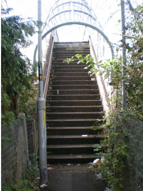
Figure 5.3: Existing Rail Pedestrian Crossings
