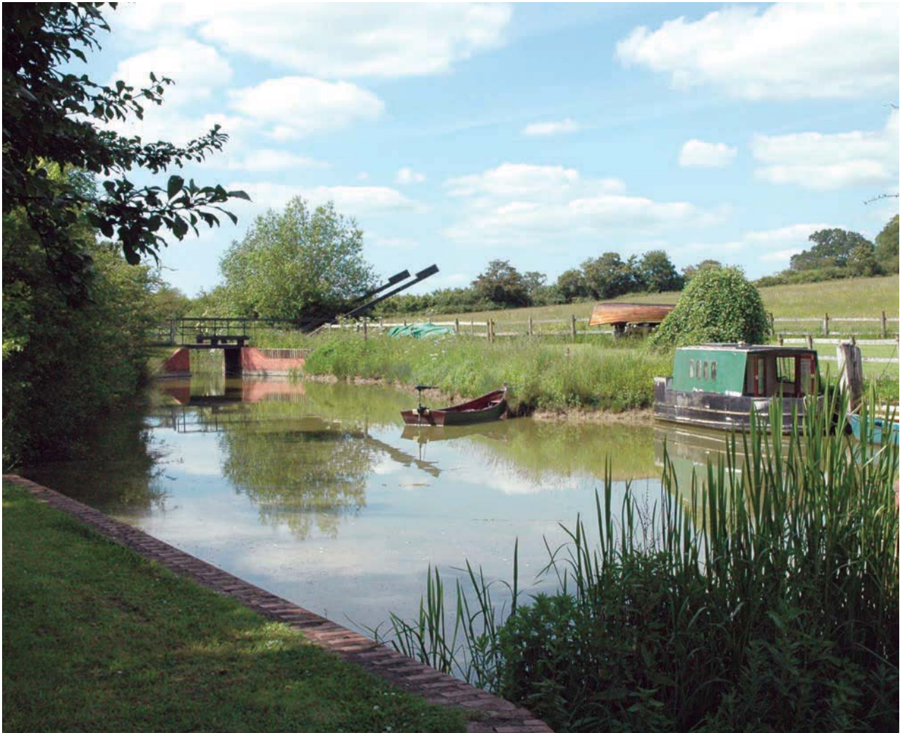
Part of the Wilts & Berks canal restored at Foxham Lock.
