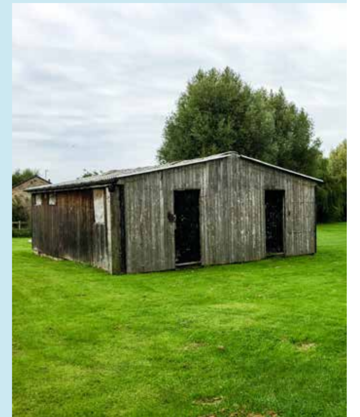
Wooden changing rooms at the Moot Lane football ground
