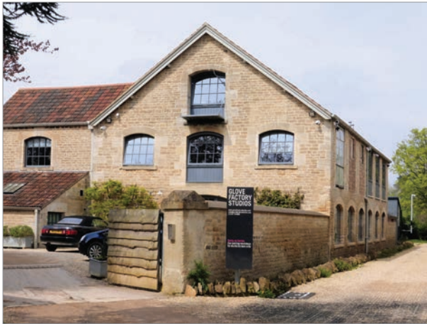
The Old Glove Factory redevelopment
