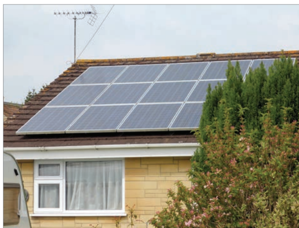
Solar panels in Holt
