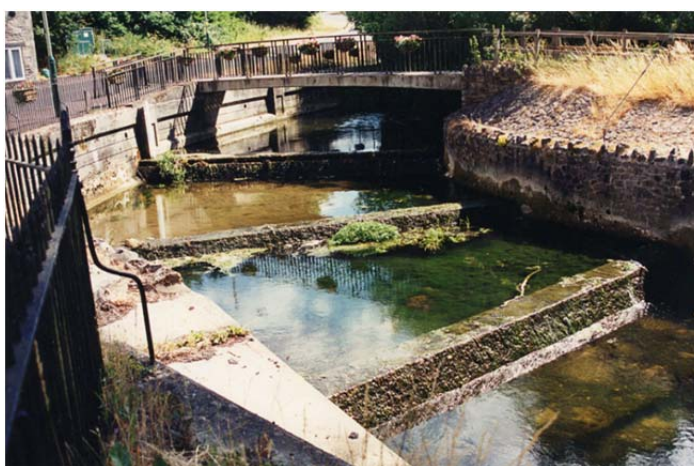
Figure 4-6: Sherston Avon at St John's Bridge June 1995
