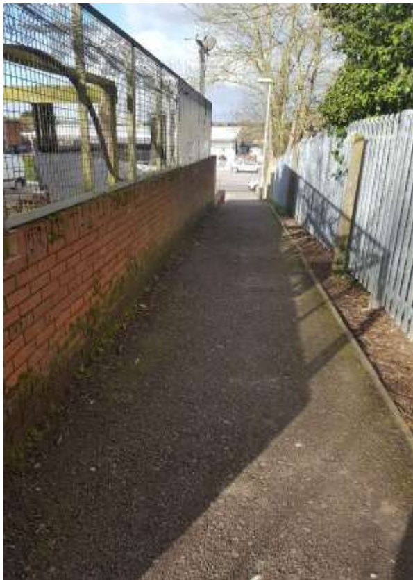
Photograph 1 – Looking north towards Andover Road
