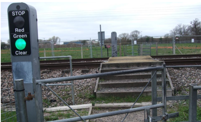
Level crossing is unaltered
