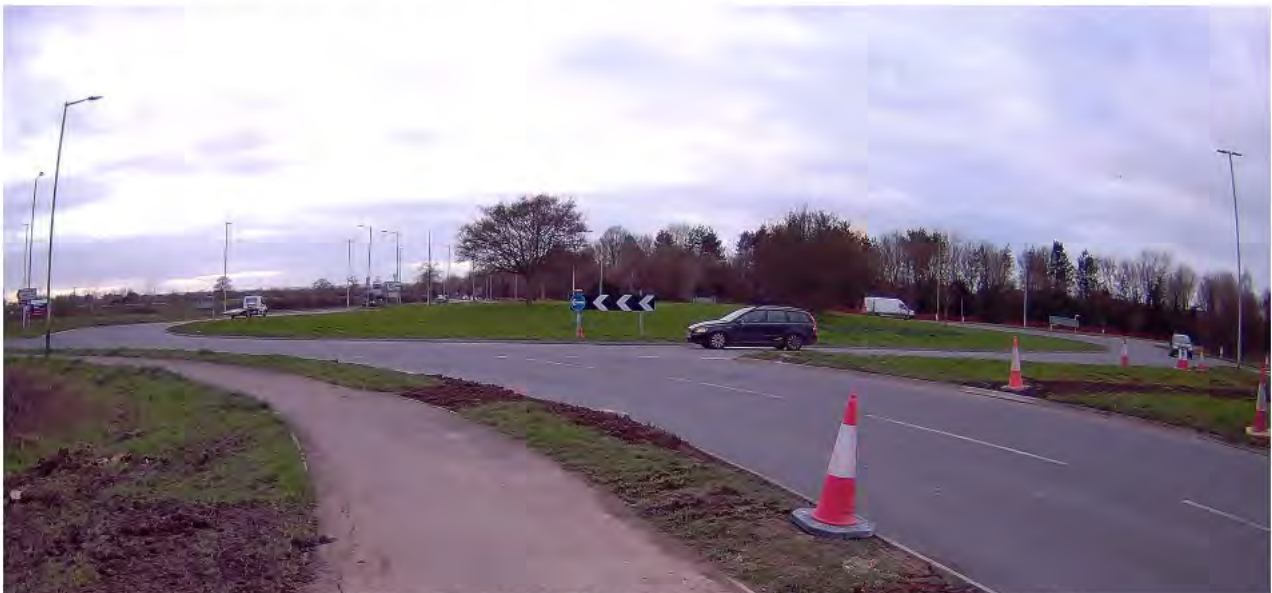
(View 4 – Bowerhill roundabout from A365, Pathfinder Way to left, Spa Road to Town, right.)
