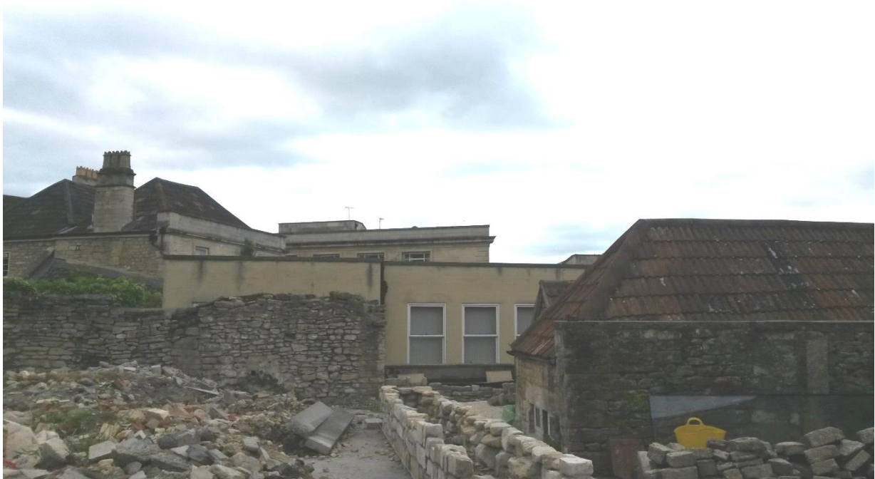
Photo from rear of No. 24 Silver Street that would face new roof addition and stairway
