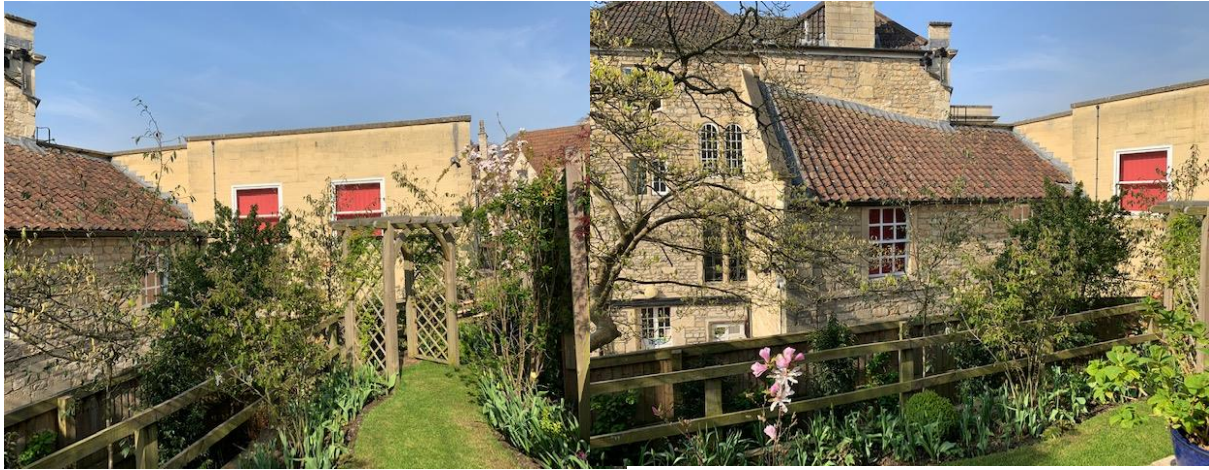
Photos from rear garden of No. 6 Mill Lane towards existing NE and N elevations of Mansard House
