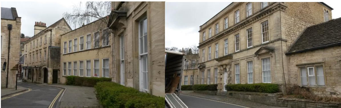
Photo of modern 20th century addition - Manvers House
