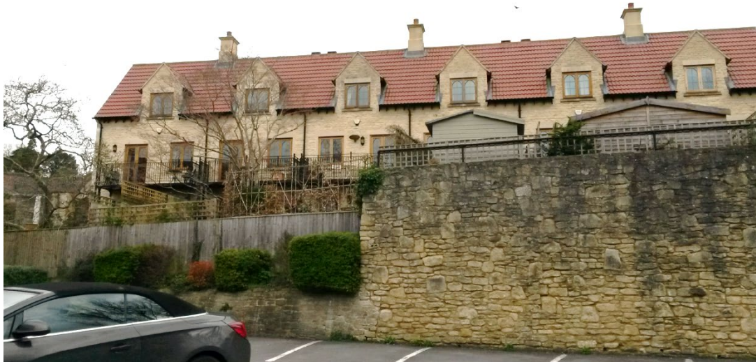
Rear of 1-6 Mill Lane
