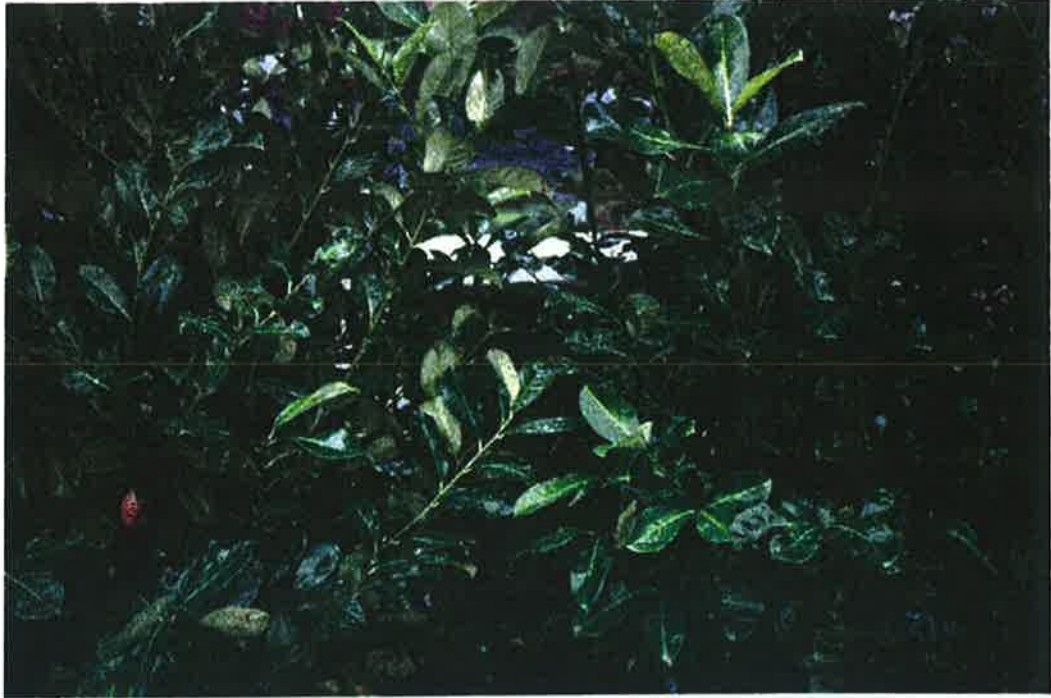
The junction box is already obscured by new growth.
