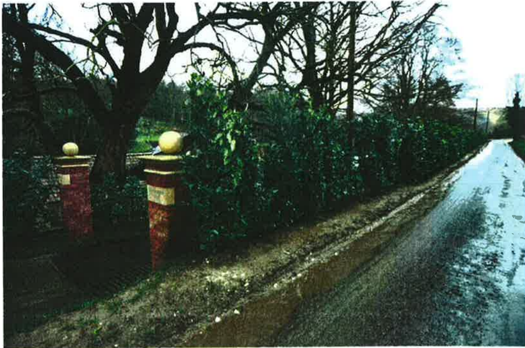
Visibility back up the road is now obscured. And also any vehicle exiting Luccombe Mill.
