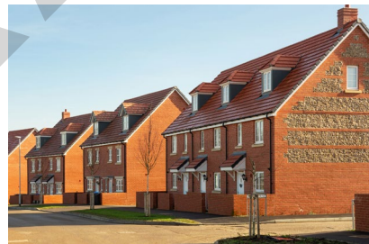
The Fugglestone development in Salisbury, which is held in the Fund's impact affordable housing portfolio
