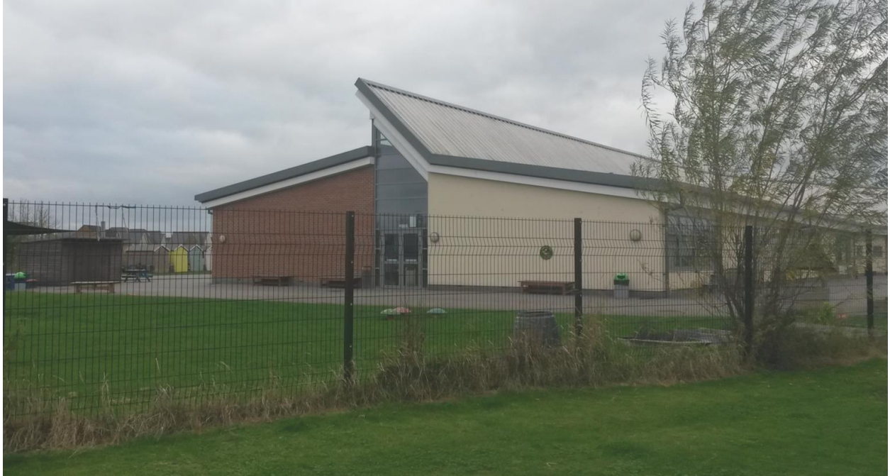
Existing eastern elevation of main building
