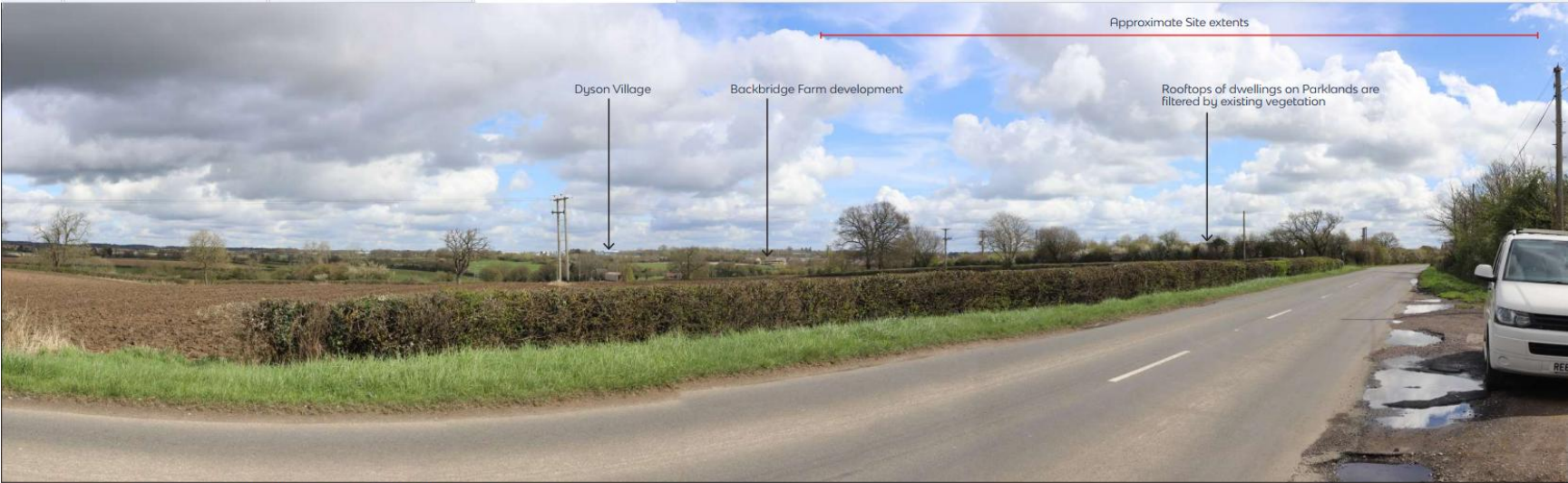
Photoviewpoint 1: View from B4040 Sherston Road looking east towards the Site
