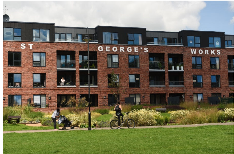
St George's Works development, Trowbridge
