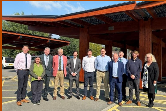
Solar car park at Five Rivers Health and Wellbeing Centre, Wiltshire Council
